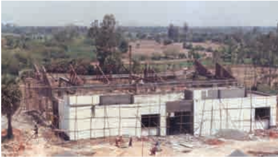
ASAN MEMORIAL COLLEGE OF ENGINEERING AND TECHNOLOGY (AMCET) - CONSTRUCTION PHASE
